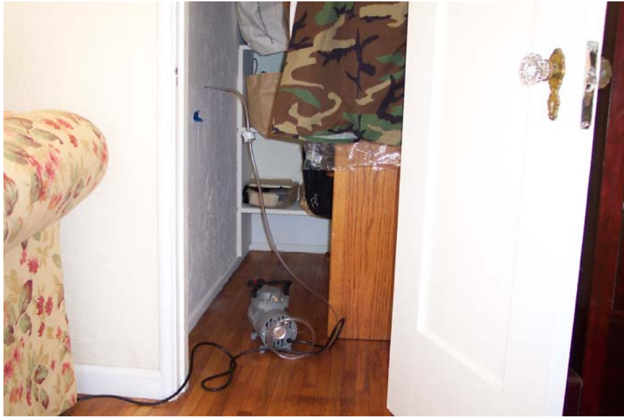
Figure 4. Digital image of wall check sample taken from closet of northwest bedroom.
