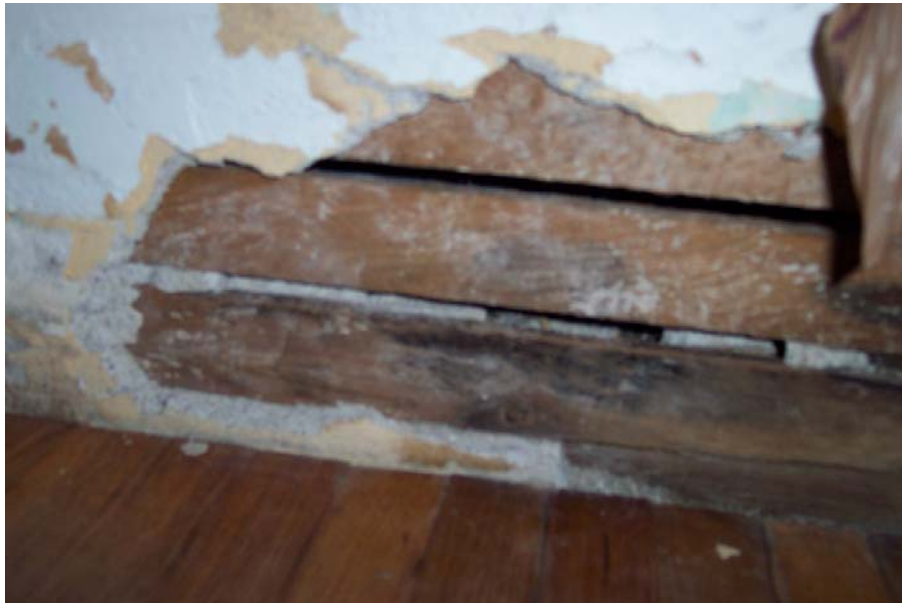
Figure 3. Digital image of area of removed drywall in master bedroom.
