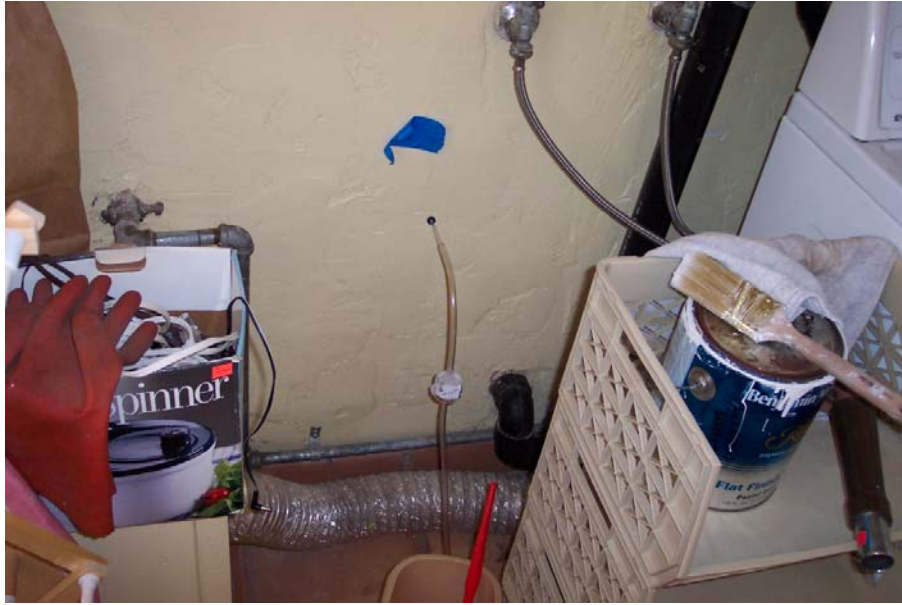
Figure 1. Digital image of laundry room wall, showing sample location.
